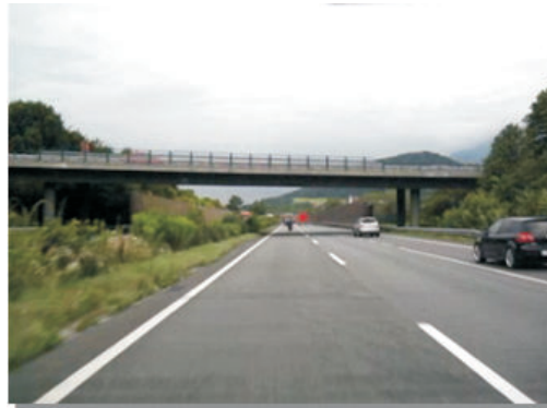
Figure 6.6: Bridge (overpass Wattens Bahnhofstrasse), driving direction east
