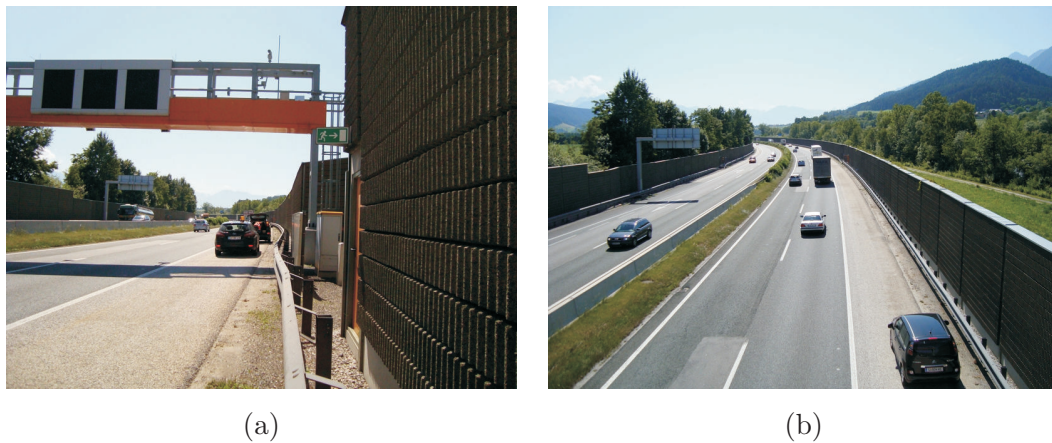
Figure 4.19: (a) Low RSU gantry and vicinity and (b) view from the low RSU gantry in direction west
