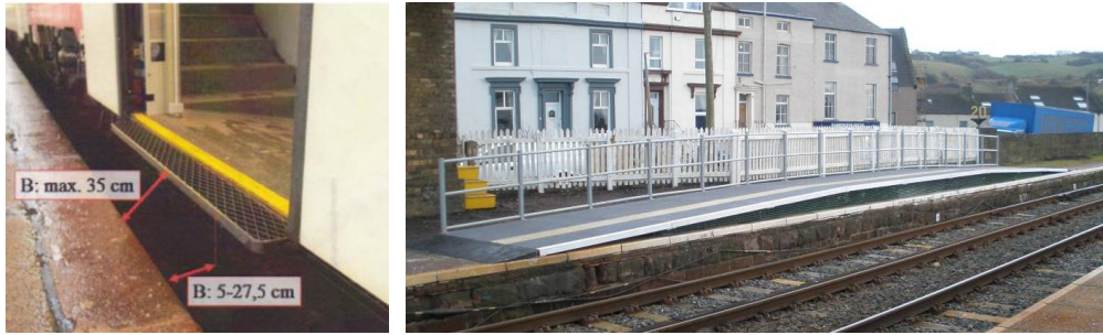
Pic. 78: vertical gap and diagonal distance (left), “Harrington Hump” (right)
