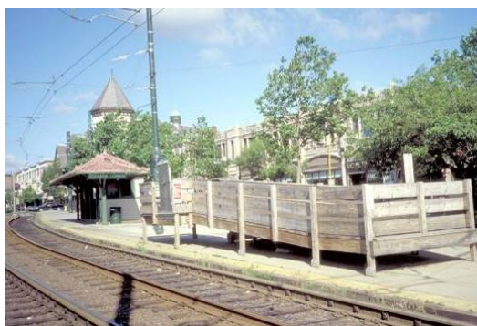
Pic. 40: permanent platform-based ramp - USA
