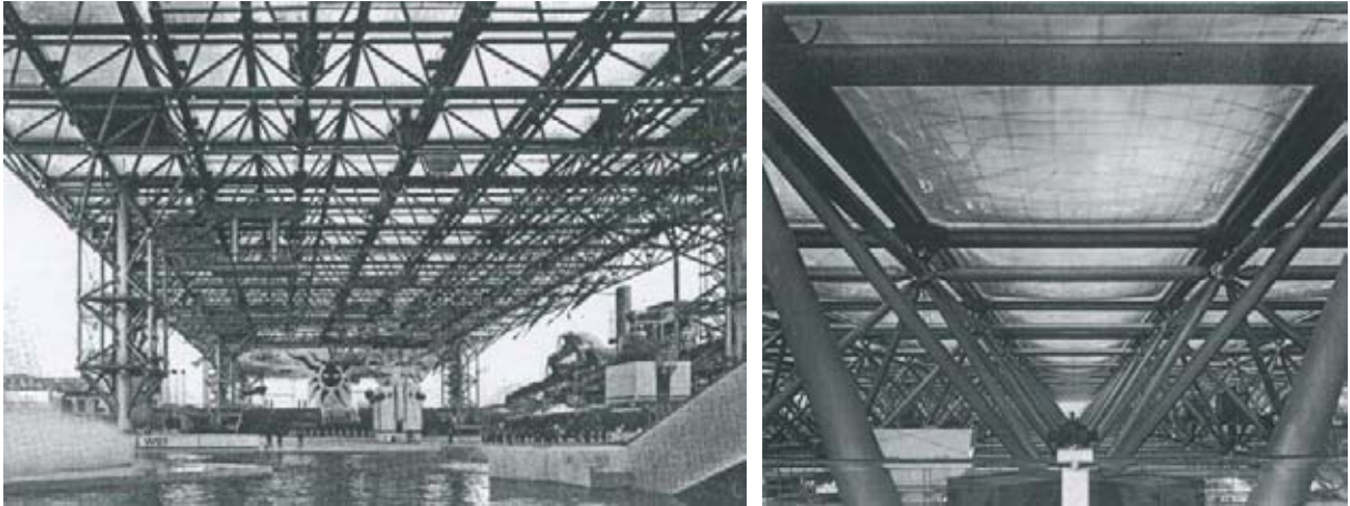
Figure 40: Space grid structure and its half-octahedron repeating units
