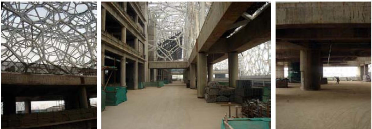
Figure 30: Reinforcement substructure of the Water Cube
