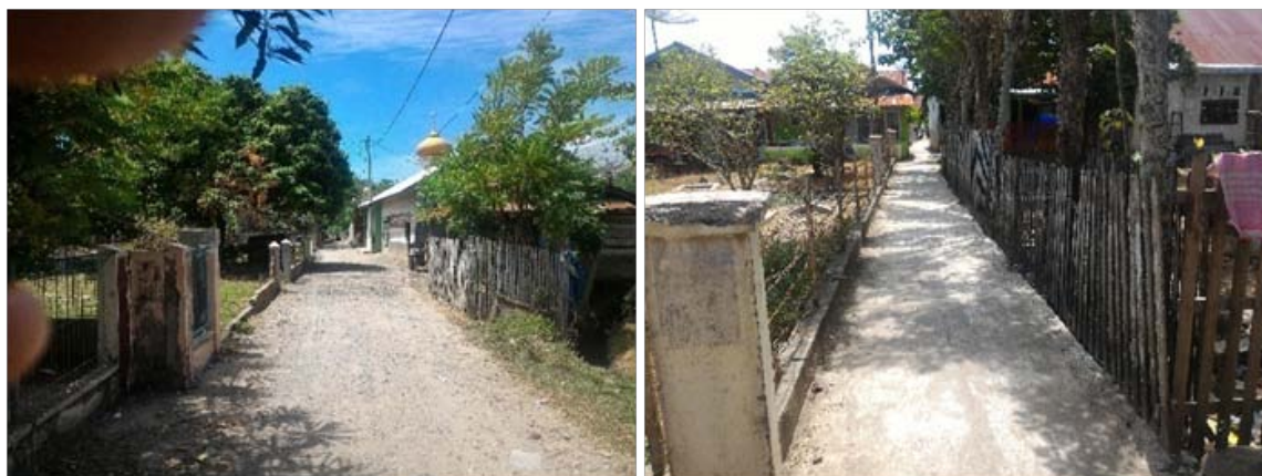
Figures 6. Roads conditions at settlements area (Source: Authors' document).
