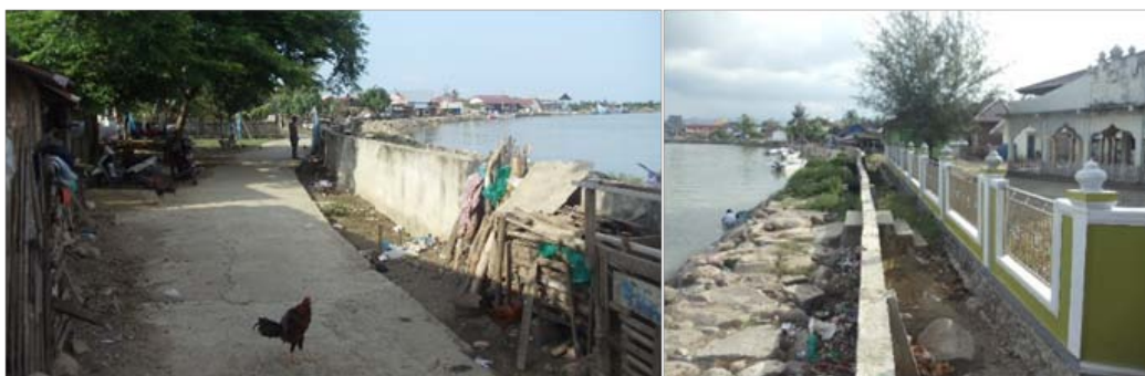
Figures 5. Inspection roads along the riverbanks. Source: Authors' document
