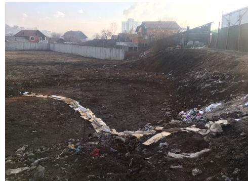
During construction. Large amounts of debris has been removed.
