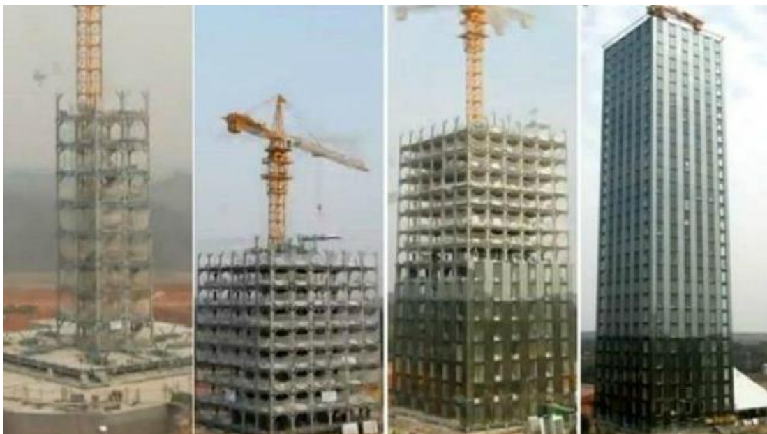
Figure 1: 30 story building which was built in 15 days in Hunan Province, China (photo source: http://freshadda.com/images_adda/30-STOREY-BUILDING/ )
