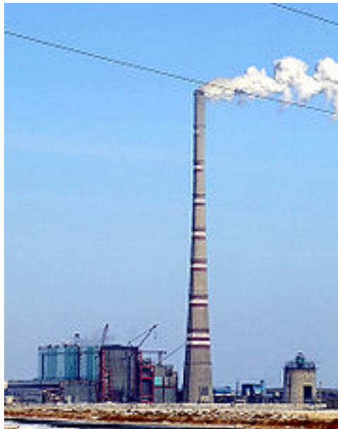
Figure 7.7: A smoke stack releasing exhaust fumes to the atmosphere.
