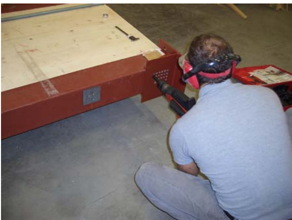
Abbildung 13: Montage eines Stahlschuhes mittels Hilti-Schussnägeln Figure 13: Assembly of the steelshoe with Hilti shooting nails
