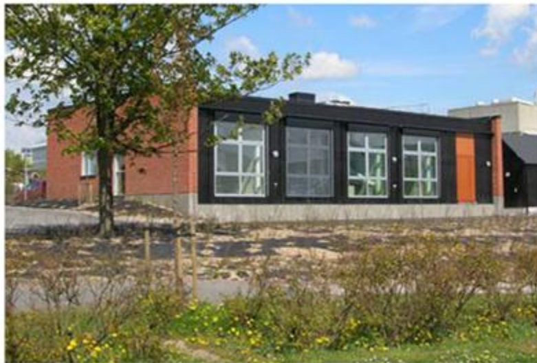
Figure 3: South facade of the LTH- system [4]
