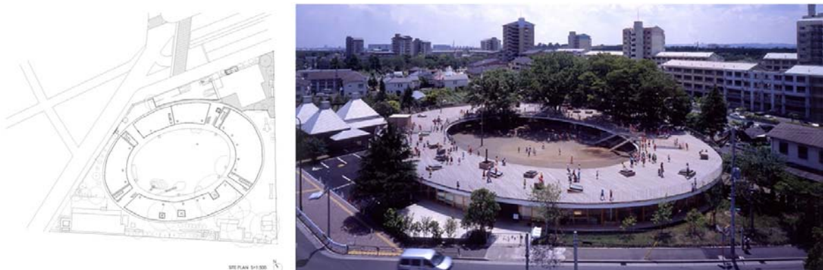
Fuji Kindergarten, Tokyo, Tezuka architects, 2007
