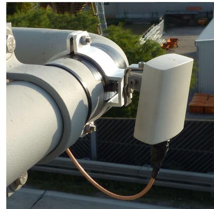
(b) RSU antenna mounted at RSU2.
