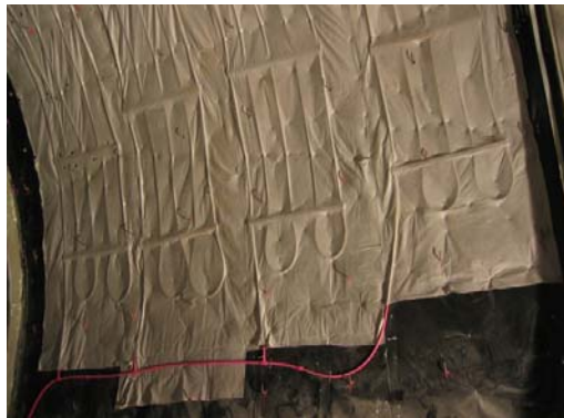
Figure 3. Detail of the four absorber loops with collection pipe (Adam & Markiewicz, 2009).
