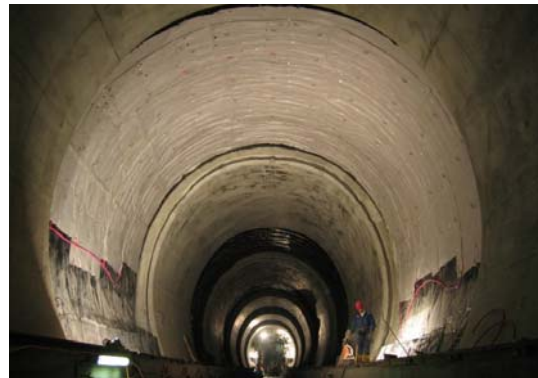
Figure 4. Energy geotextile at lot LT22 of the Lainzer tunnel (Adam & Markiewicz, 2009).
