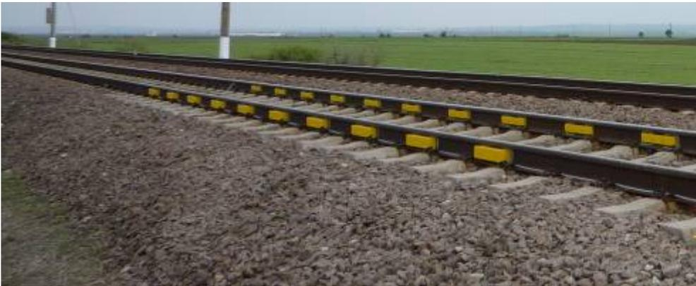
**Figure 2.** Axle load checkpoint G2000 at Zimmnitsa
