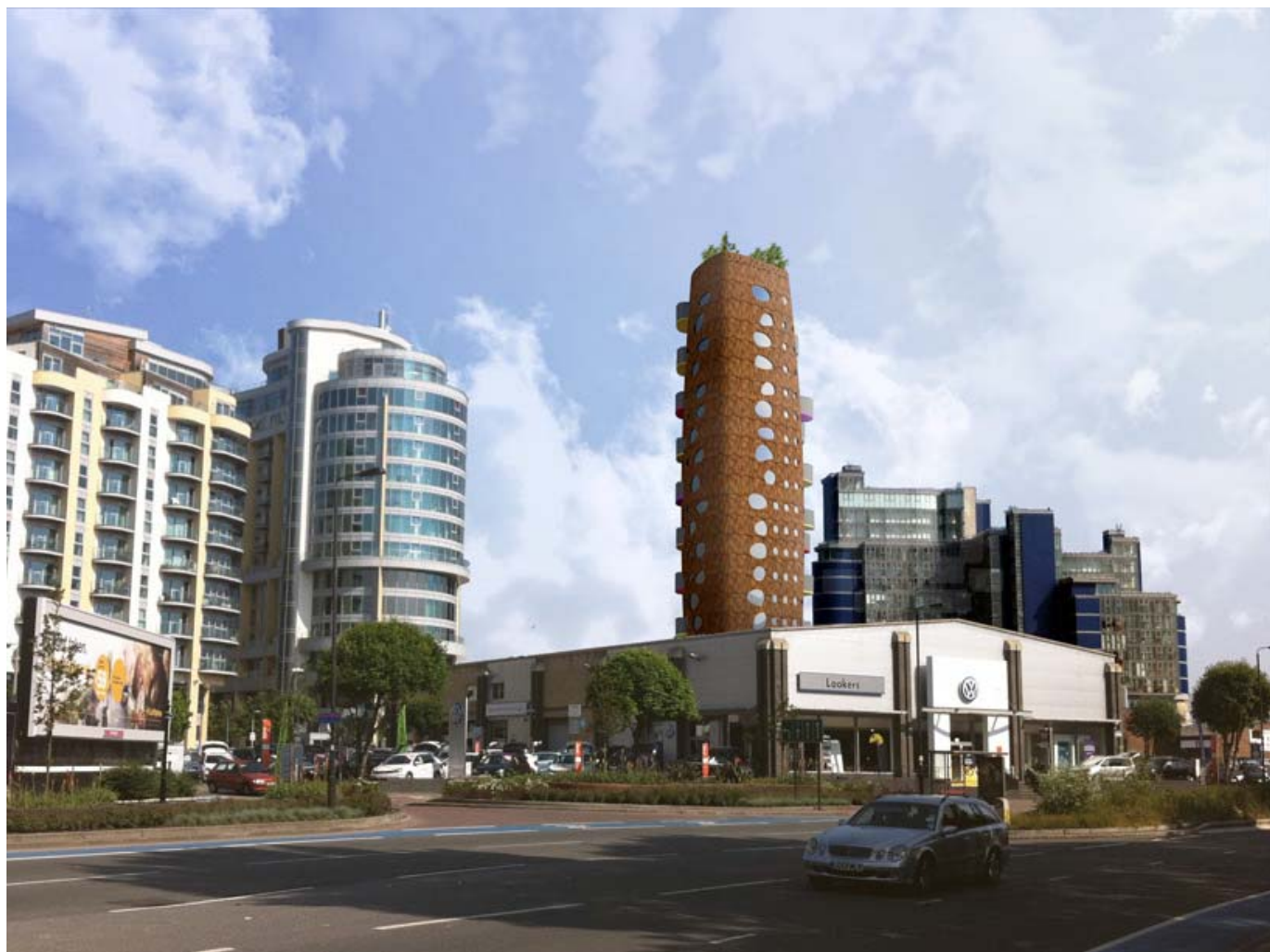
the weathered steel provides a reddish brown coloration, in contrast to the urban context
