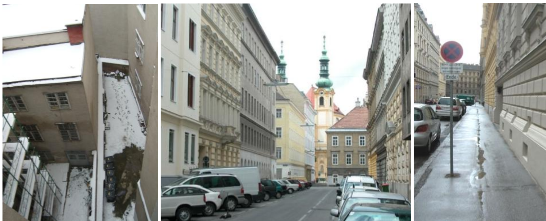
Fig. 3: obstructed inner courtyard - street profile in a Viennese Gründerzeit quarter – narrow sidewalk.
