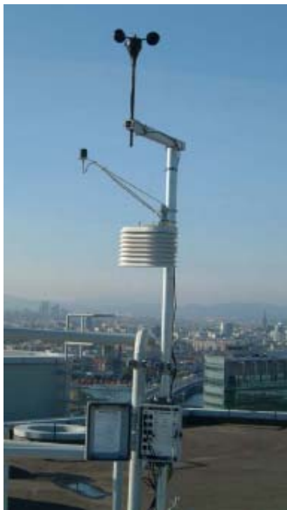
Figure 14: Weather Station mounted on the roof
