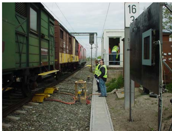
Figure 7: Test train on May 10 th , 2005 at the Checkpoint prototype: System for monitoring the train gauge and for the detection of fire.
