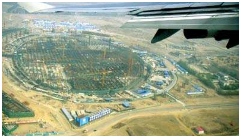
Pic. 3: Construction close to Beijing Airport in 2005 in Germany construction areas bare, uncovered soil and accumulation of construction waste are exposed to wind, leading to regional sandstorms and soil deflation.
