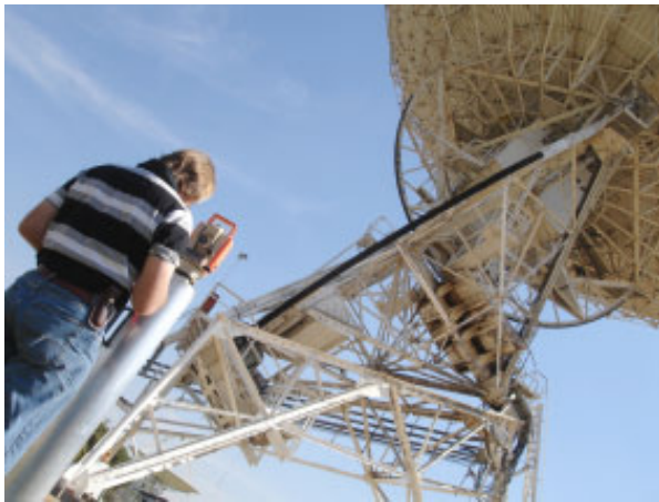
Fig. 2 Ludwig Combrinck surveying the 26m's polar shaft during bearing repair (Credit: Mike Gaylard).
