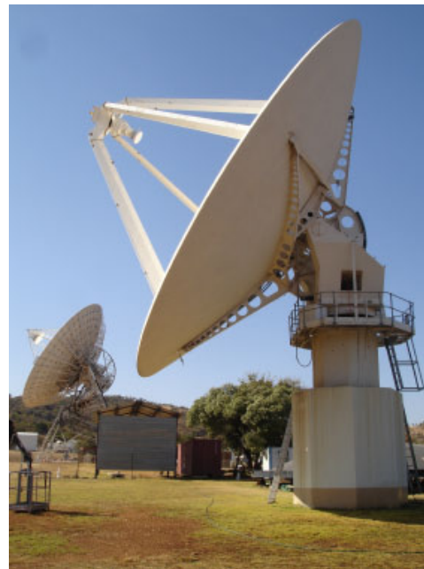
Fig. 4 HartRAO 15m telescope mount with offset elevation axis (Credit: Mike Gaylard).
