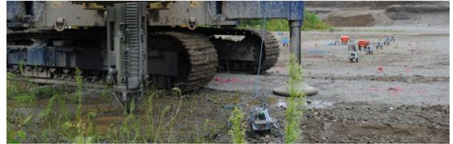
Figure 7. High sensitivity accelerometers on the ground surface to record ground accelerations.
