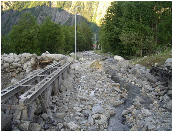
Figure 51: Example of deposition of debris on a regional road caused by the outburst of a water pocket of Rochefort glacier
