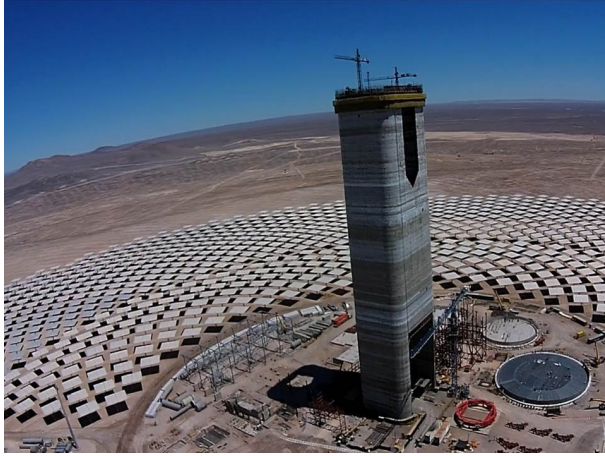
Figure 1.1.: Picture of the construction side of the 110 MW Cerro Dominador CSP plant in Chile with storage tank basement in 2019 [121]
