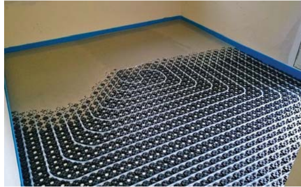
Figure 2.21: Radiant floor installation, courtesy of Novelec [58]. Tubes circuit and insulation surfaces are visible under the cement layer
