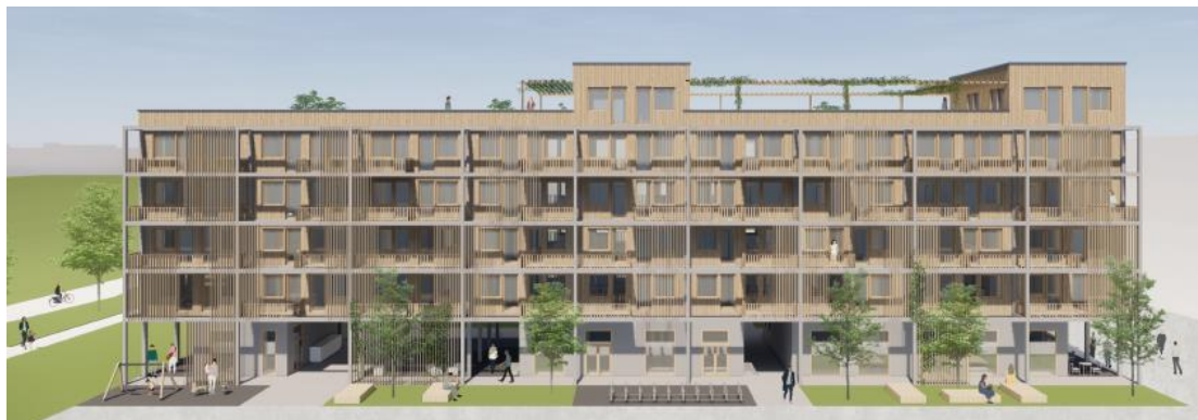
Figure 2: Pilot Case, Project example BAUM home
