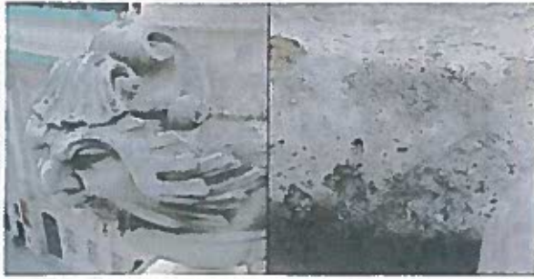
Figure 3: Sandstone decoration on the roof of the Hofburg (Vienna, AT): the slurry is being pushed away from below by fungi and lichen growing out of the pore space.
