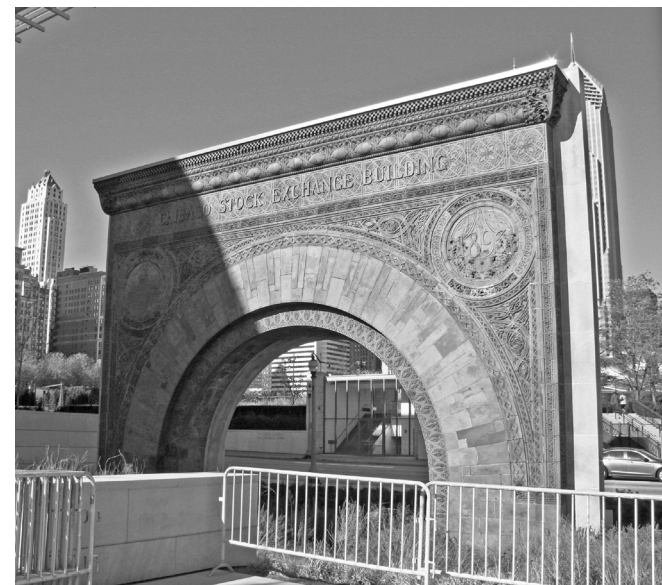
Abb. 2: Chicago Stock Exchange , Chicago, IL, 1893-1894, Louis Sullivan, Eingangsbogen
